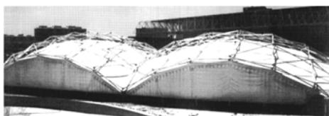
**Figure 7:** Deployable swimming pool cover in Seville, Spain[28]
