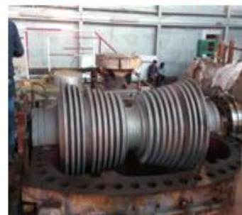
IP Turbine Dismantling
