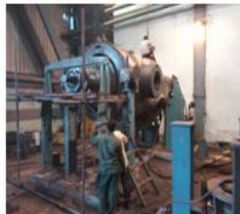
HP Turbine dismantling
