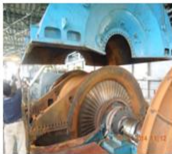
LP Turbine dismantling for inspection
