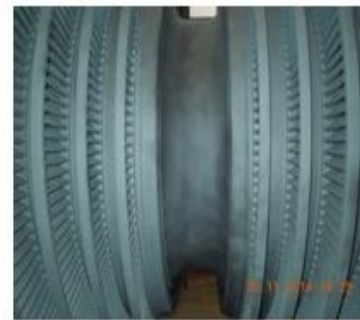
Turbine Rotor after Alumina Blasting
