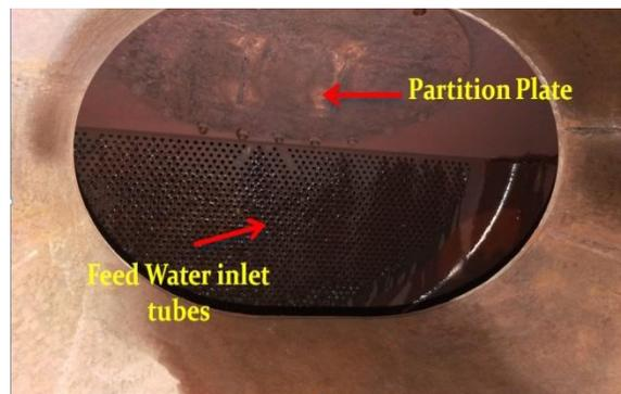
Fig.6: View of water tubes in heater
