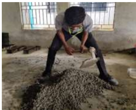
Figure 4. hand mixing of concrete
