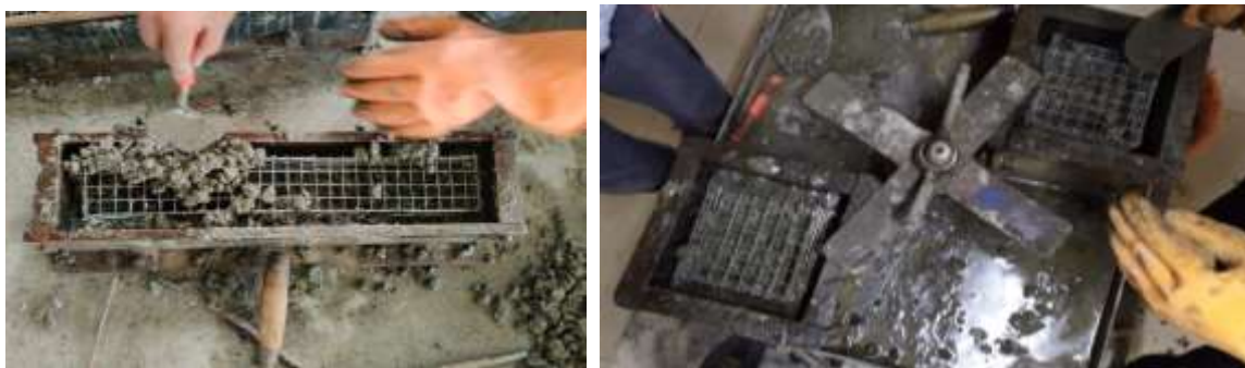
Figure 6. placing of concrete in moulds with steel wire mesh.
