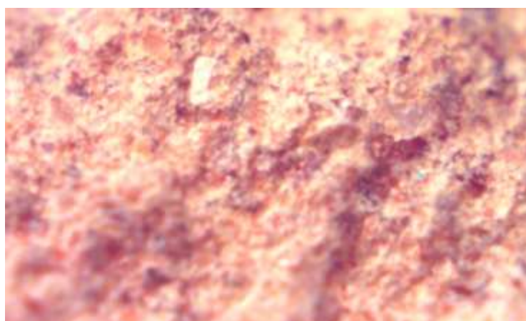
Figure 9: The structure (x100) of a sample of a brick of the upper part of the wall
