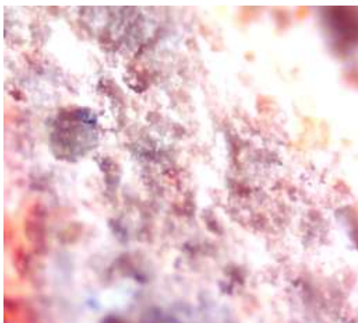
Figure 5a: The structure (x100) of the sample of the historical masonry mortar of the upper part of the brick wall of the mausoleum of Ismail Samaniy
