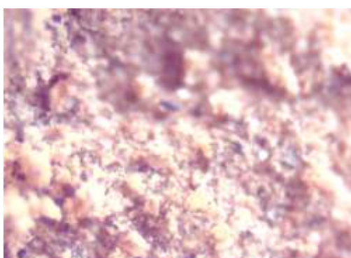
Figure 7a: The structure (x100) of the sample - samples of the historic masonry mortar wall of the madrasah of Abdulazizkhan
